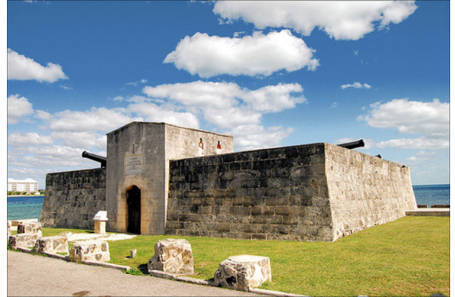
Fort Montague, Nassau, Bahamas. Completed in 1742.
